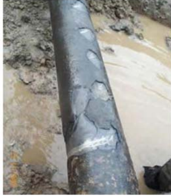
Figure 2. Pipeline coating damage due to excavation.
